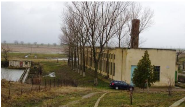
Figure 2. Pumping station building, Babadag, county Tulcea
