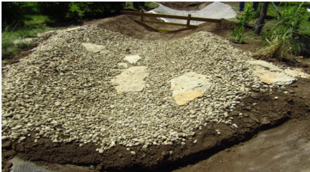
Figure 10. Channel sector finished - view
