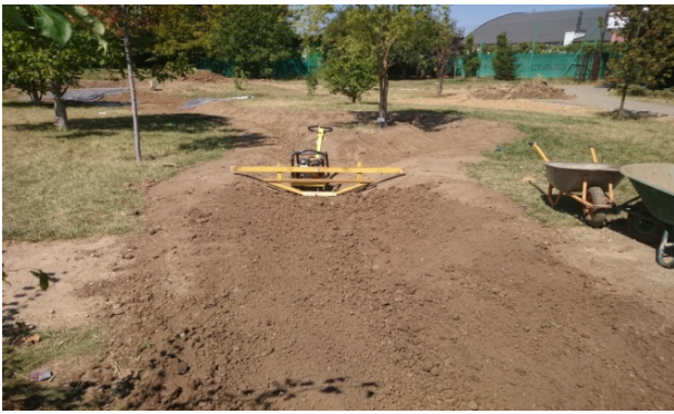
Figure 9. View of soil ready for compaction
