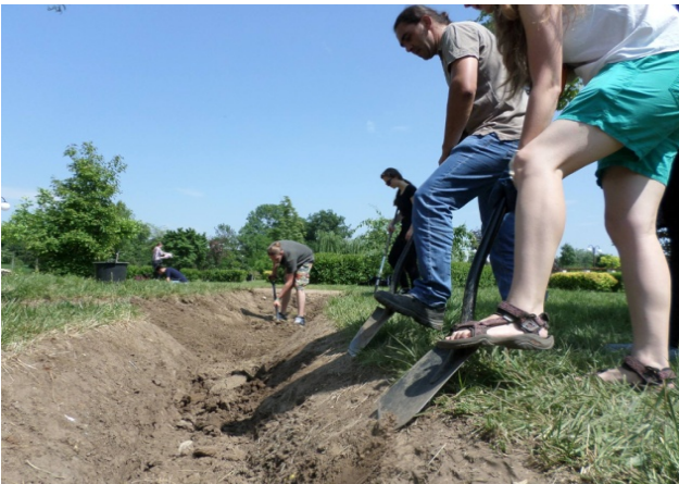
Figure 6. View within bank of ditch arrangement
