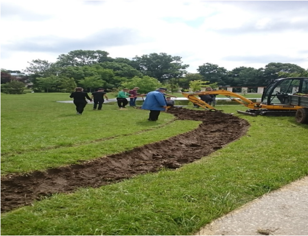
Figure 5. View within the mechanised excavation stage
