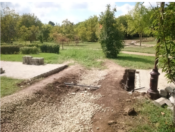
Figure 7. Bridge abutment tranche - view
