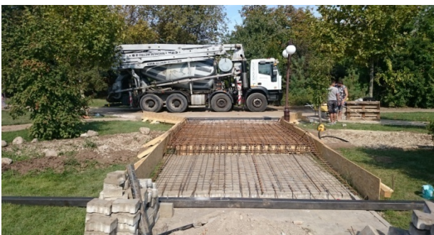
Figure 11. Preparing for concrete placement - view
