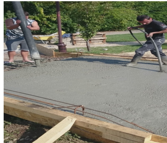
Figure 12. View of concrete placement
