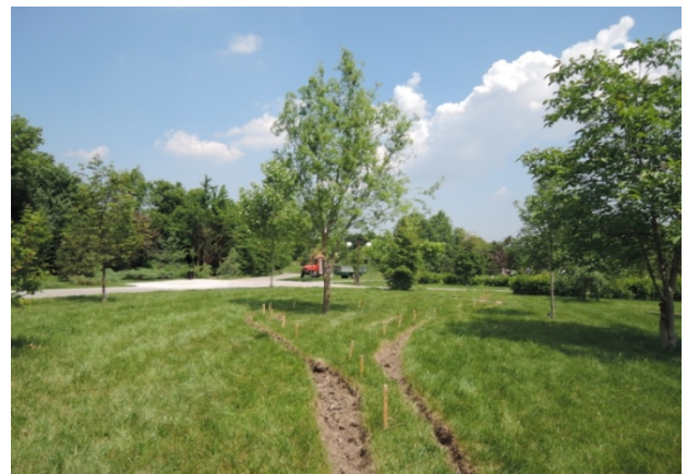
Figure 2. Channel axis – execution stage
