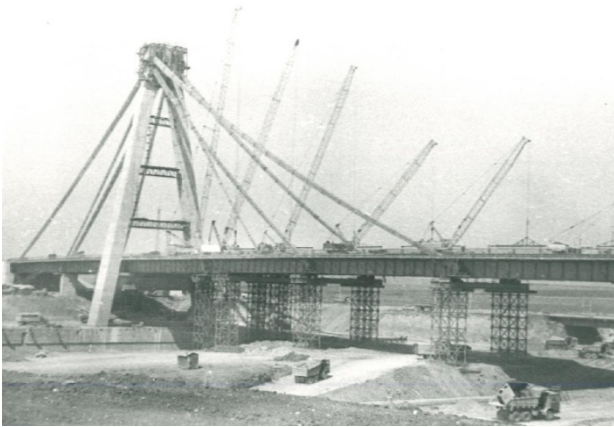
Figure 4. Construction of the bridge
