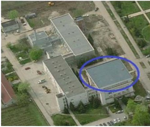
Figure 6. Building chosen for seismic assessment
