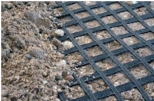
Figure 6. Geogrids covered with ballast
