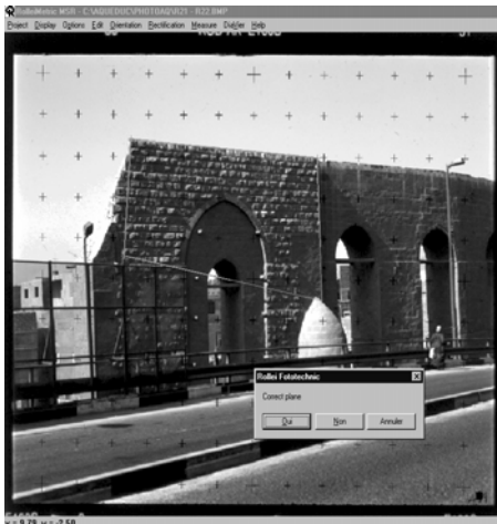
Figure 8. Building photogrammetric image.
