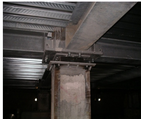
Figure 5. Example of application of base isolation method
