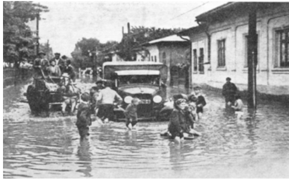
Figure 3. The effects of Colentina's drainage on Bucharest and the surrounding areas (Caranfil, 1963)
