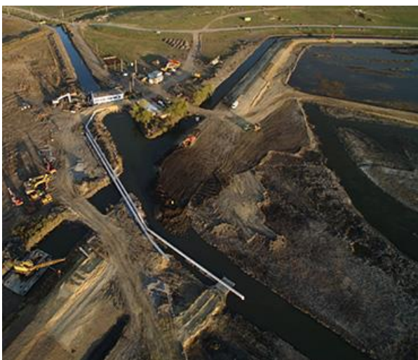
Figure 1. Works carried out in Polder Zaghen ( http://www.coralconstructii.ro/en/rezervatia-biosferei-delta-dunarii/ )
