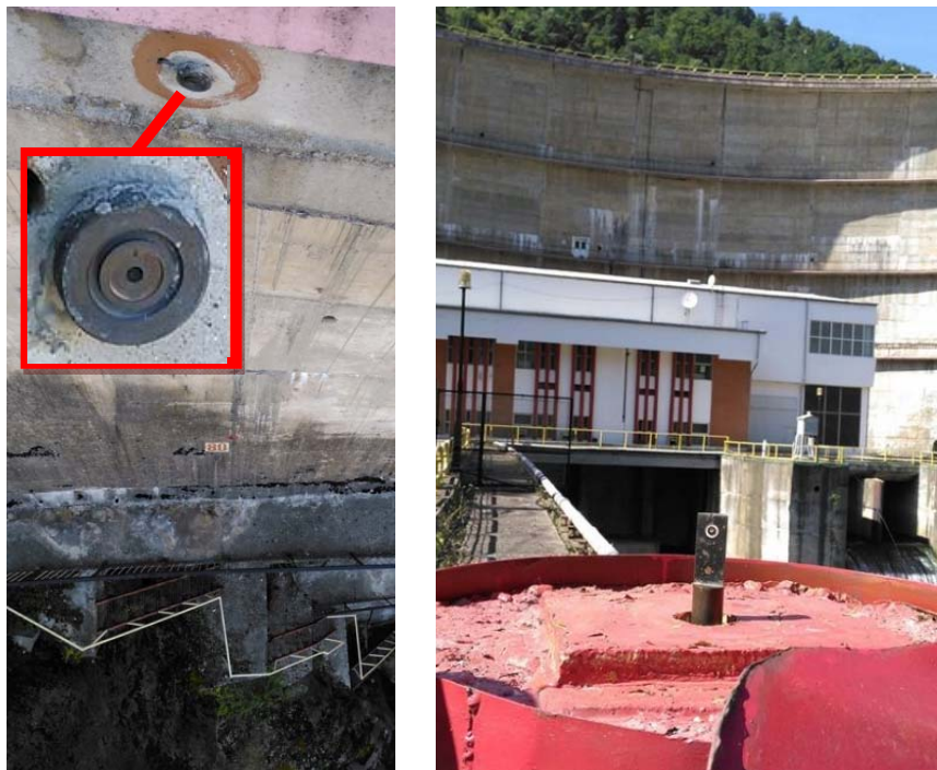
Figure 1. Survey mark and pilaster
