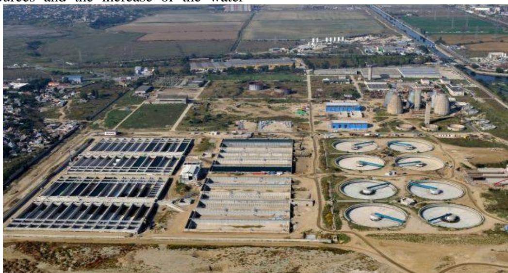
Figure 1. Waste water treatment plant Glina
