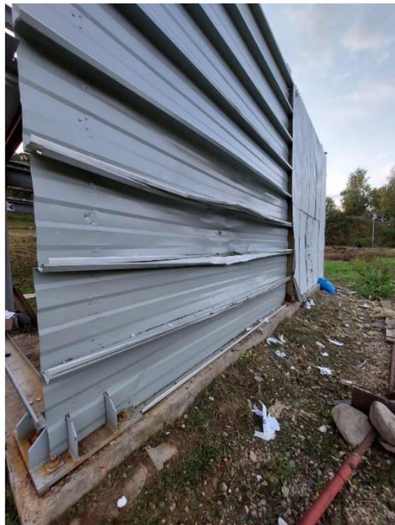
Figure 4. After-blast footage of the deformed panels
