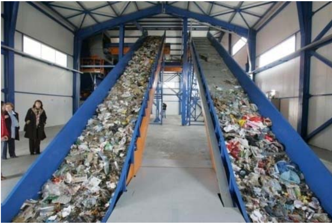
Figure 3. Waste sorting and transfer plant
