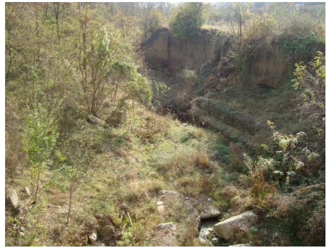
Picture no 2. Ravine shore erosion
