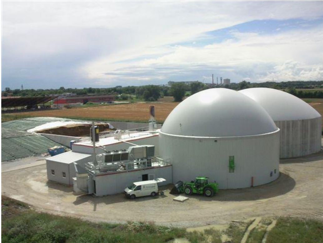
Figure 6. Biogas power plant
