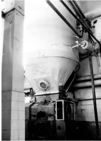
Figure 2. Pneumatic shock wave system on metallic bunker for malt viscous milling in beer plant
